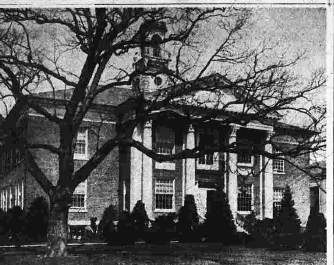
Manchester's Town Hall or Municipal Building (above) is a busy place these days. The entire basement of the building is given over for Civilian Defense use. This building looks like a beehive on a July afternoon. Manchester has 1,200 of its citizens in Civilian Defense in all departments. We are ready, boys.
